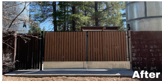
Upgrades of the wall and gate at well site
